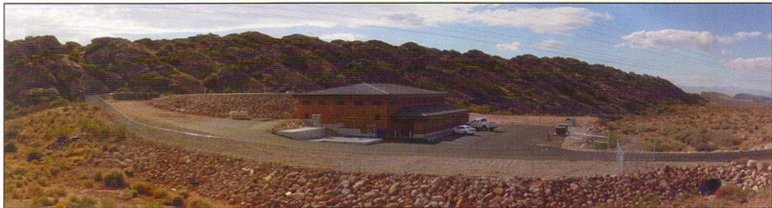
A panoramic view of the finished Microfiltration Plant
